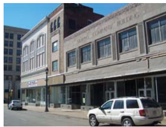
Murphy Building Before
