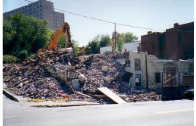
The Ellis Hotel being demolished in September 1992.
